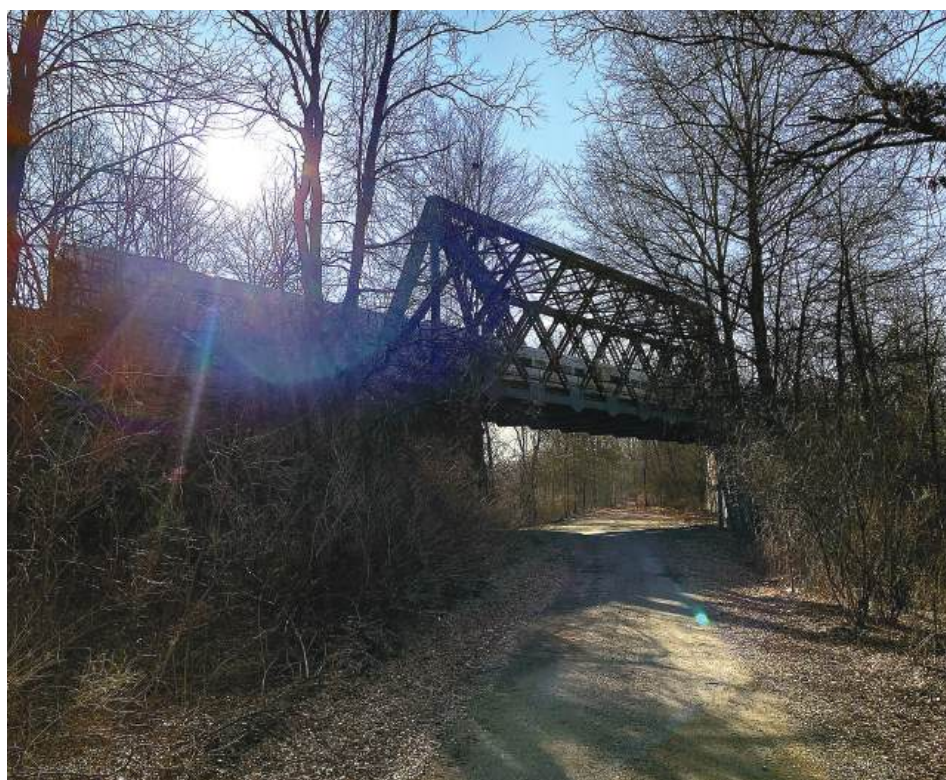
HISTORIC STEELWORK: An old steel trestle bridge that now carries Metro-North trains is easy to walk to from the parking lot in Hamptonburgh. Visitors can view trains, like this one on the bridge, from afar, but are not allowed to walk near train tracks. Luke Broge photo
