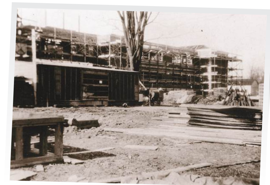
FOUNDATIONS OF LEARNING: The Washingtonville Central School building during construction, ca. late 1920s. Moffat Library photo
