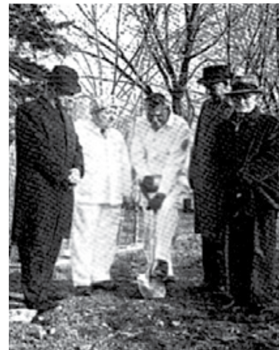
BREAKING GROUND for the construction of the BG Ambulance Corps building in 1963. The building was completed and dedicated on May 22, 1966. Photo taken from undated Orange County Post article.
